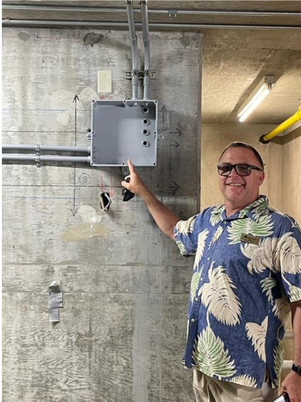
Conduit and get home Boxes being installed
