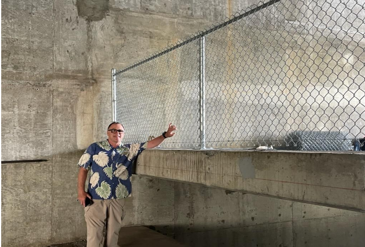
New Fencing Installed
