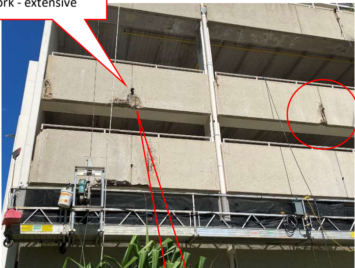
Paoakalani Spall work in progress
