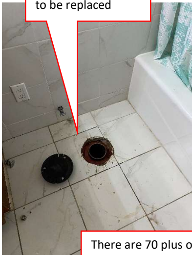
Typical toilet flange to be replaced
