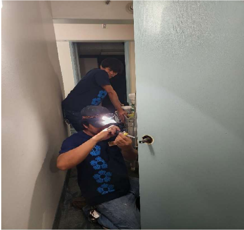
Tower 2 37 th Floor Trash Room Door Maintenance
