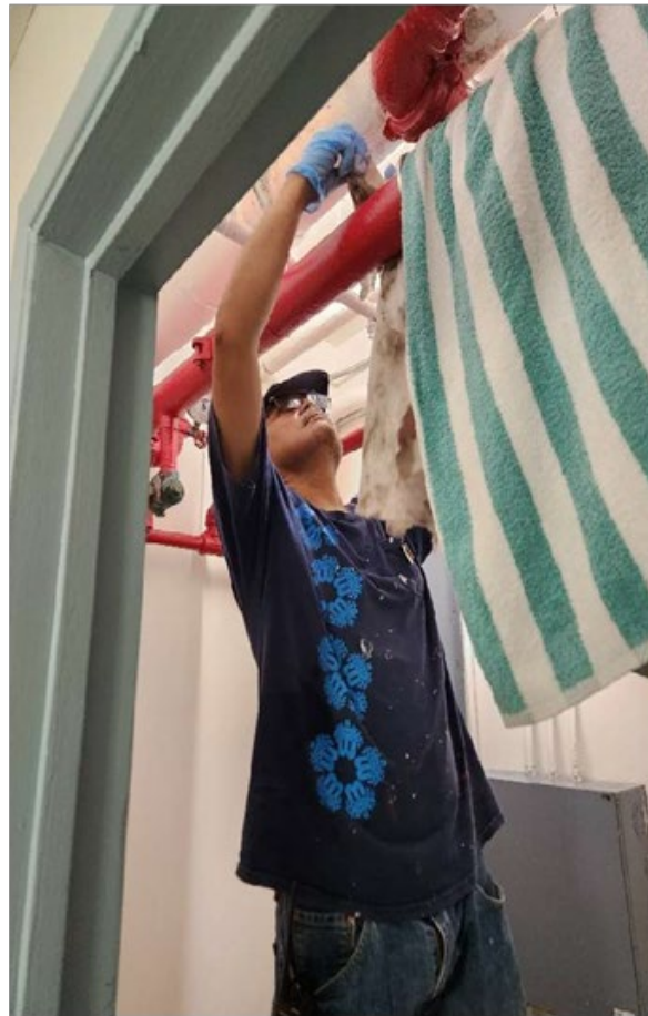
Fire Sprinkler Safety Repairs
