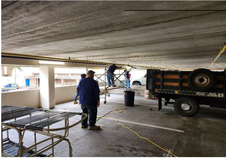
Replace Vent Pipe Tower 2 nd Floor
